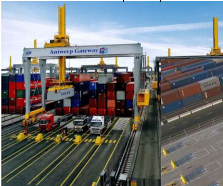
Gate/ rail Interface (trucks)
