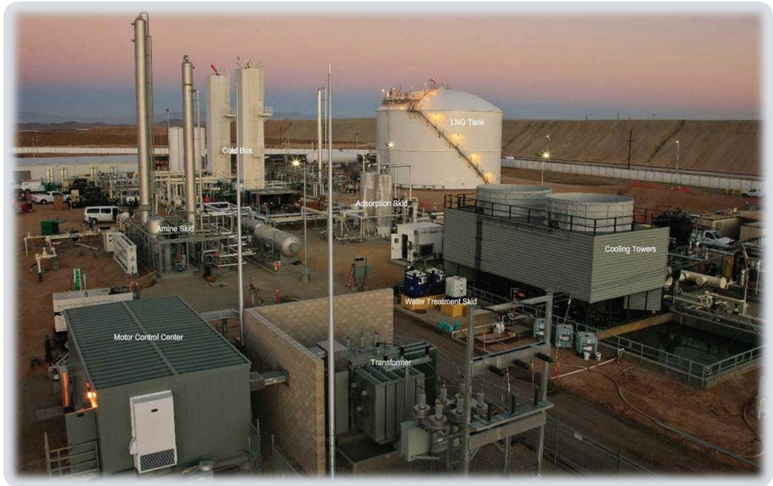
Clean Energy's Boron, CA 160,000 gpd LNG Plant – Located on 15 acres
