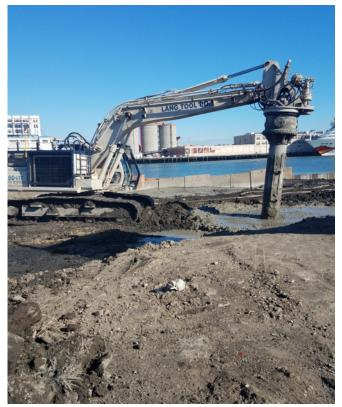
FIGURE 10: In-Situ Concrete Stabilization Operation
