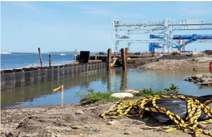
FIGURE 8: Bulkhead Installation at Coastal - 2018
