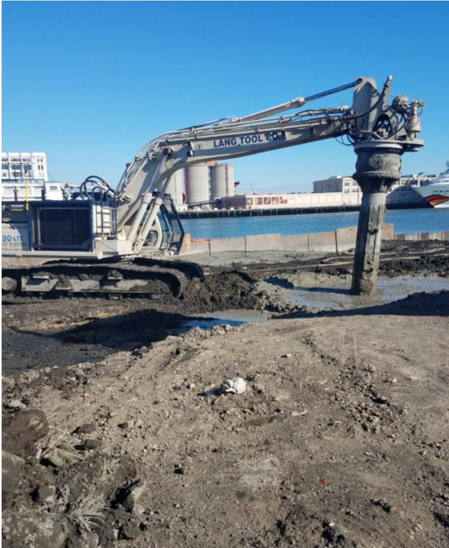
FIGURE 10: In-Situ Concrete Stabilization Operation
