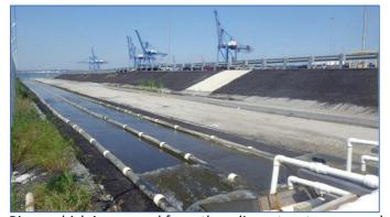
MDOT MPA originally partnered with the University of Maryland to develop the system and Maryland Environmental Service to operate it. The AFT is a linear raceway constructed at the Dundalk Marine Terminal (DMT) located on the Patapsco River (Figure 1-1). The AFT uses water from the Patapsco
